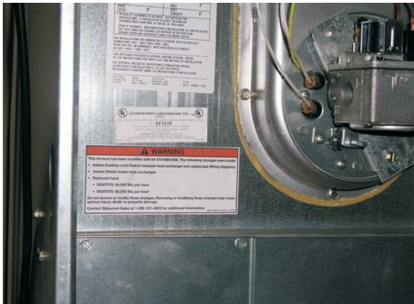
FIGURE 31: Install warning label directly below rating plate on vestibule panel.
