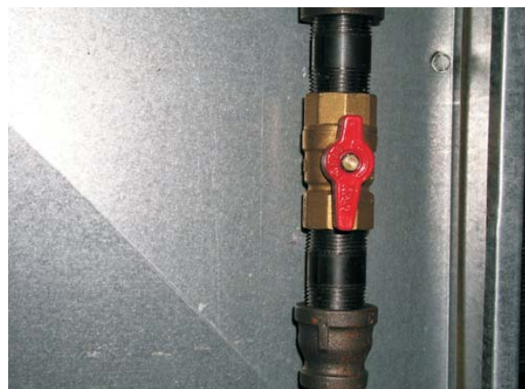
FIGURE 48: Turn gas supply back on and leak check gas valve piping connection.
