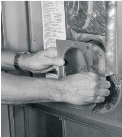
FIGURE 14: Remove burner chute mounting screws (4) and remove burner chute.
