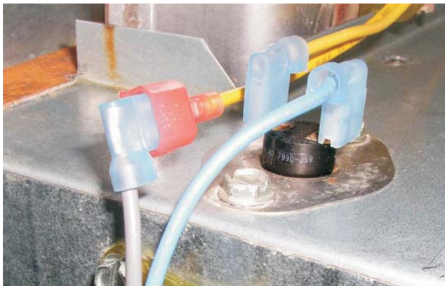
FIGURE 44: Install new auxiliary limit switch leads in series with upper limit per wiring diagram.
