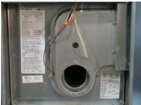
FIGURE 11: Remove pressure switch tube.
