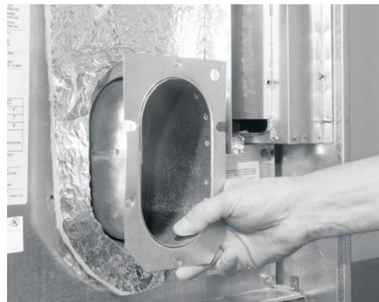
FIGURE 24: Reinstall burner chute to original position.
