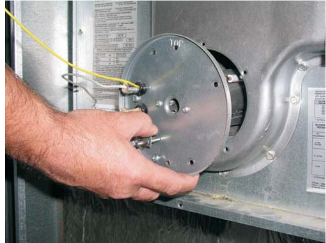
FIGURE 28: Reinstall burner.
