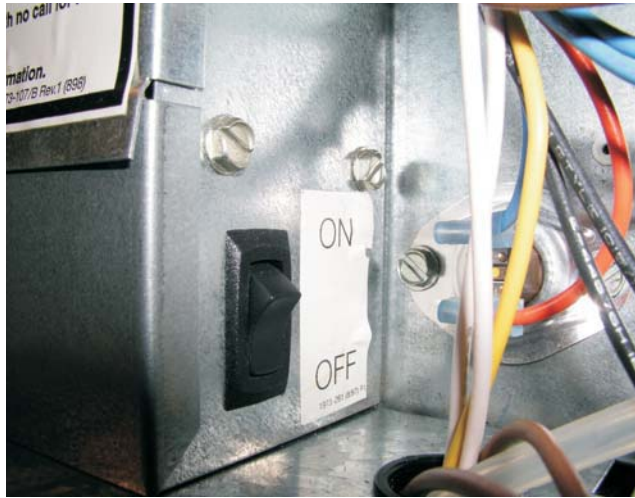
FIGURE 49: Turn electrical back on.
