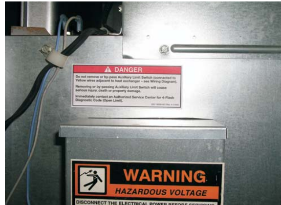
FIGURE 47: Install danger label on vestibule panel just below upper limit switch.
