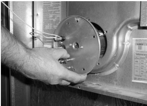
FIGURE 4: Burner assembly removal
