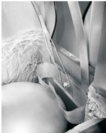
FIGURE 38: Compress stainless loop in middle to slide past heat exchanger. Do not skin or scrape foil from insulation while sliding switch down side of heat exchanger.
