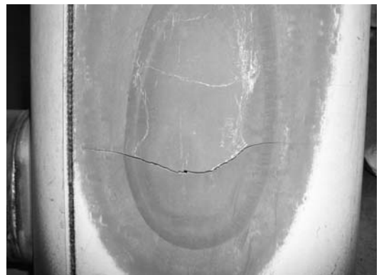
FIGURE 7: Cracked heat exchanger
