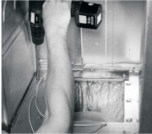
FIGURE 43: Install new wire clamp in blower shelf hole on rear left-hand side of shelf. Reinstall (7) screws to secure blower shelf.
