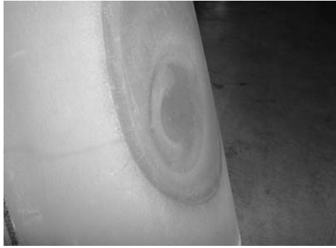
FIGURE 8: Deformed heat exchanger
