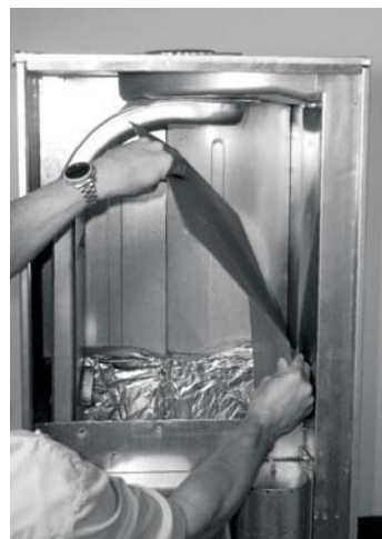
FIGURE 36: To protect side wall insulation insert cardboard sheet as a "shoe horn" to insert auxiliary limit switch assembly between insulation and heat exchanger.
