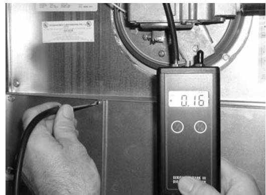
FIGURE 52: Measuring supply static pressure
