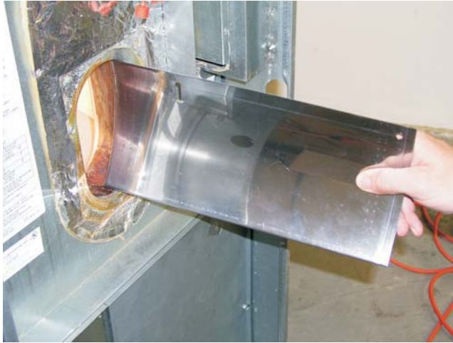
FIGURE 19: Insert Part B and rotate upwards.
